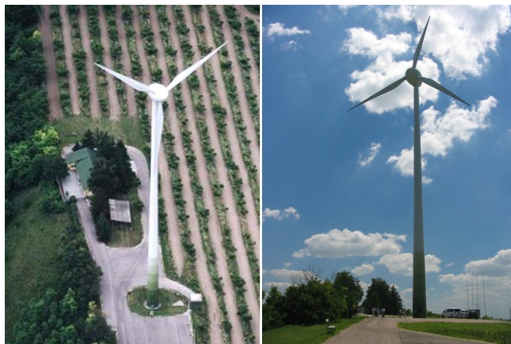
Wind generator in Kulcs
